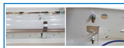
Drill hole on gear tray to secure the lamp clip
